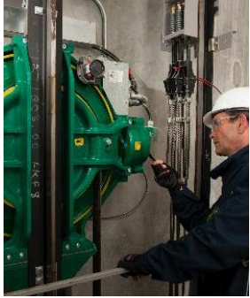
1996 KONE MonoSpace® machine-room-less elevator
